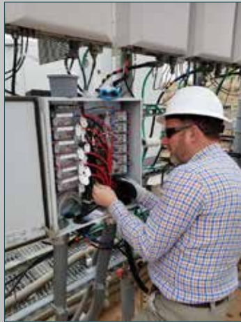
A technician terminates DC power in a Raycap Inverter
