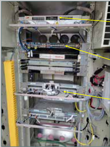
PDU or DC Power Distribution Unit
