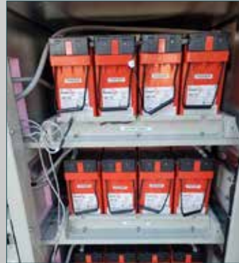
24 VDC Batteries
