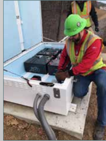
An electrician installs a backup battery system for highway lighting
